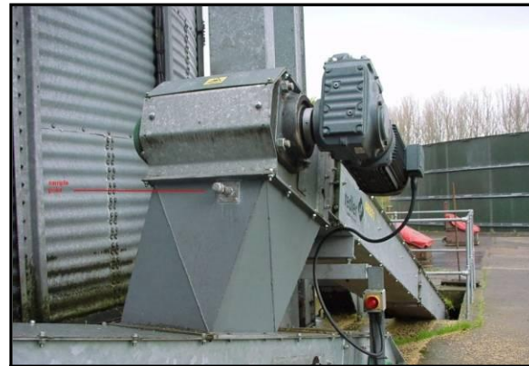
Crisp- Intake 4 Conveyor
